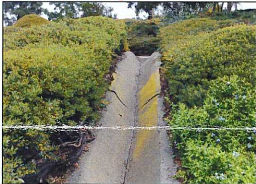
cracked V-ditch
